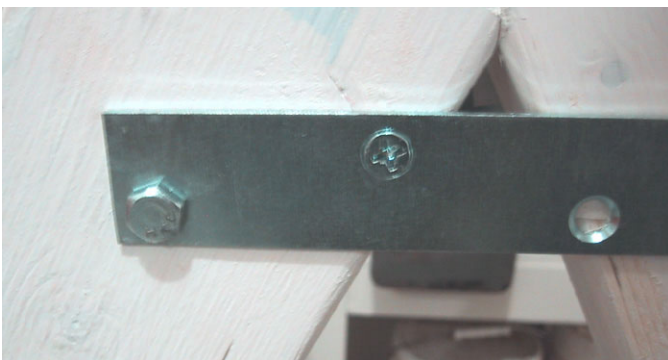
Photo 10. Close view of left side of the hinge.
